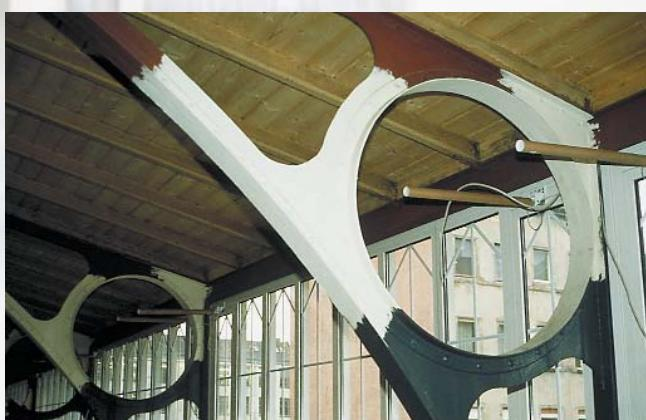
All primed surfaces must be clean, dry and free from dirt and grease etc. Mechanical damage must be made good with approved priming system before application proceeds. PROMAPAIN<sup>®</sup> must be applied in accordance with the manufactures instructions and care must be taken to ensure the specified dry film thickness is achieved.
